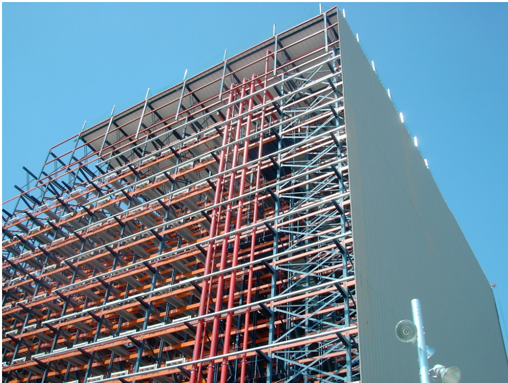
Figure 8, Rack storages can be fitted in existing buildings, new buildings made for it or rack structures can be covered with wall and roof elements (rack supported building).
